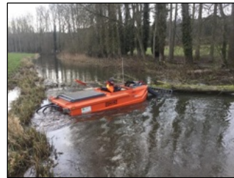
We carefully remove blockages from rivers to prevent flooding and avoid disturbing wildlife.
